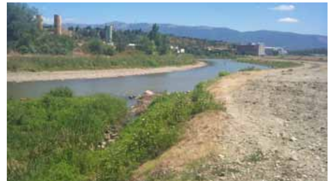
Image 19. Existing open storm water canal
